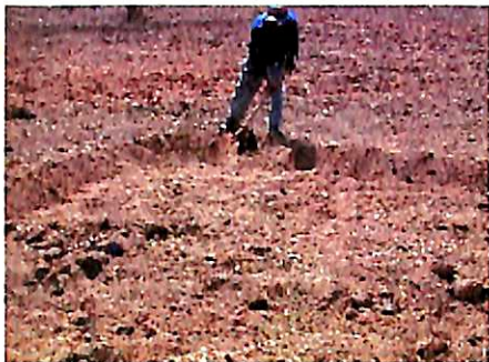
Left : Construction of a V-shaped micro-catchment in the field
